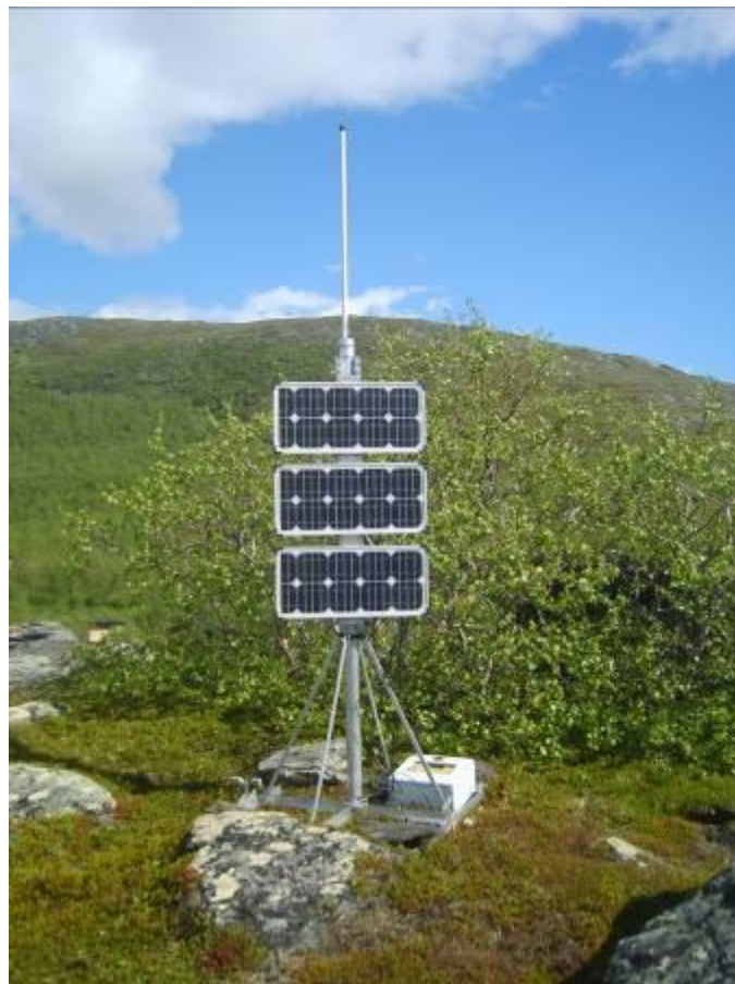
FIGURE 30 SOLAR PANEL AND STAND WITH ROUTER
