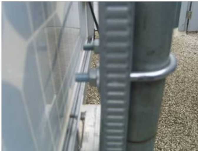
FIGURE 28 SOLAR PANEL MOUNTING HOLES BRACKETS
